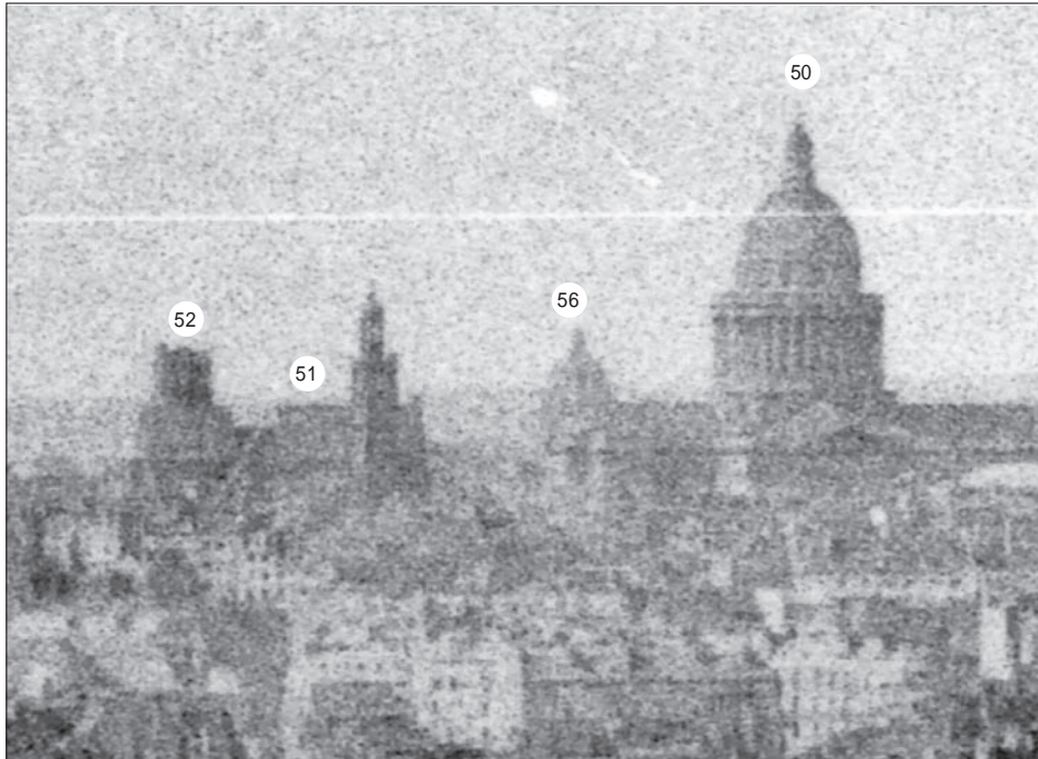
C10 Roof of Saint-Étienne-du-Mont, detail of photograph, Fig.106
